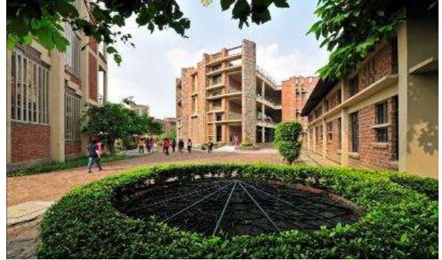
Rainwater harvesting System and Sewage Treatment Plant
